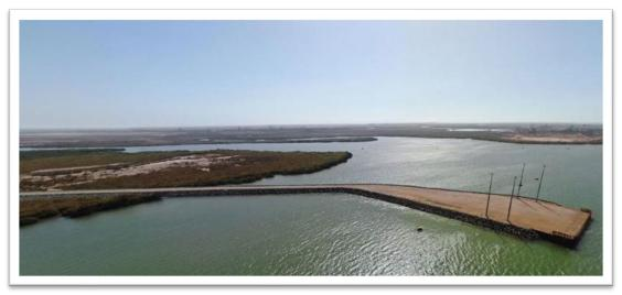
Work has started at Lumsden Point to construct the seawalls, which will be followed by widening of the causeway to the wharf.
